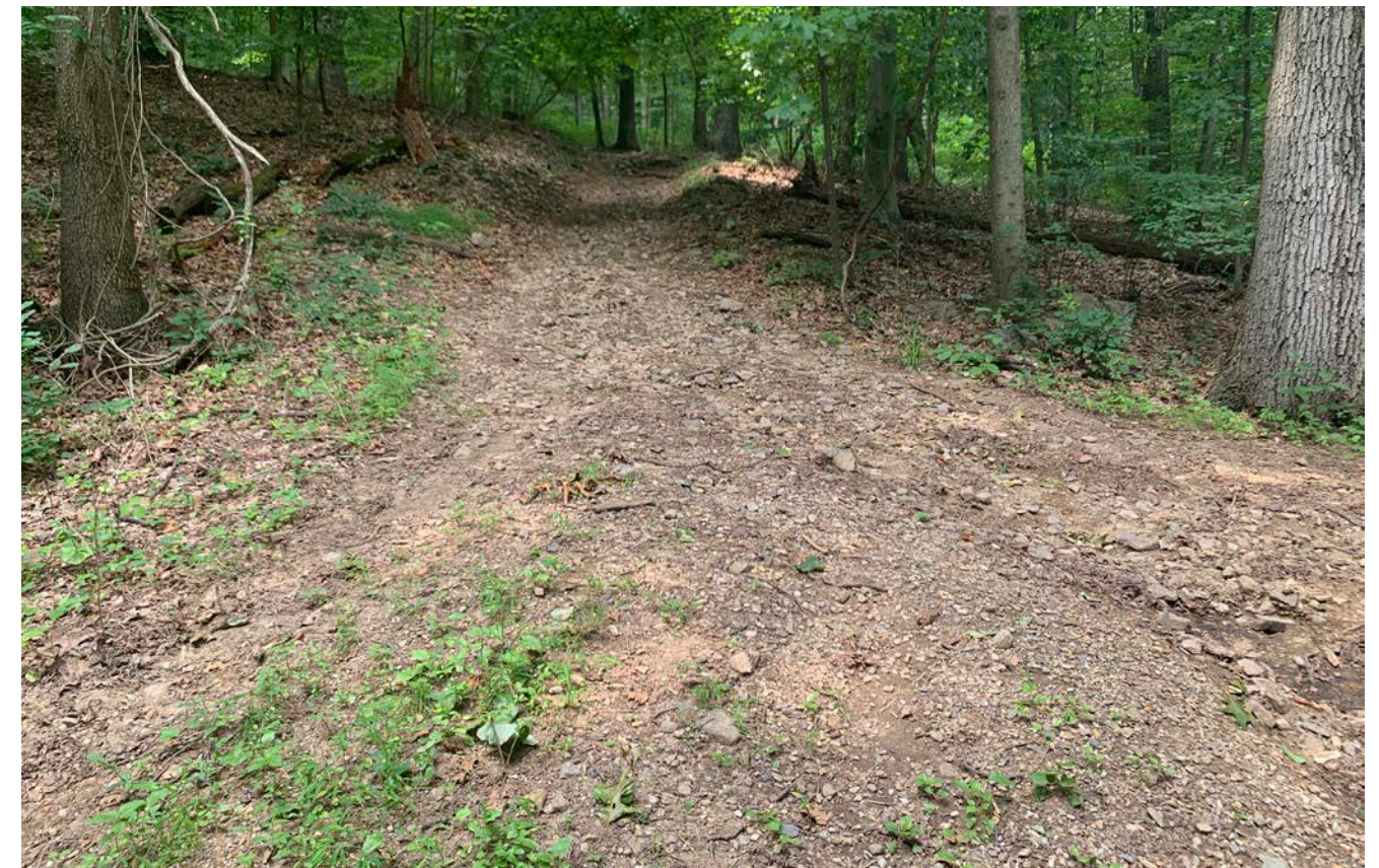
Steep trails frequently erode more quickly, as water travels more rapidly along steep trail surfa.
