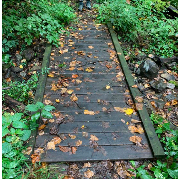
An example of a small footbridge crossing a shallow channel.
