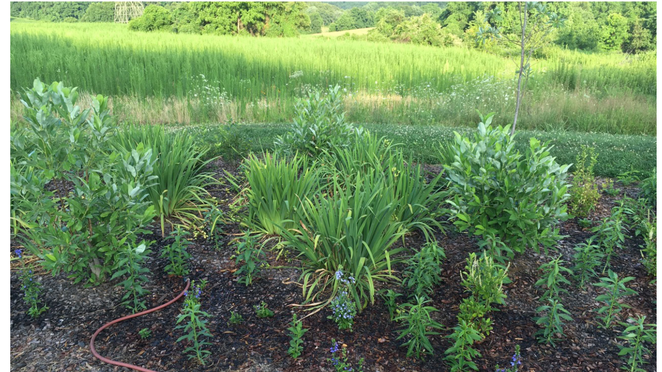
Stormwater can be captured in swales or rain gardens. Photo: Dan Barringer
