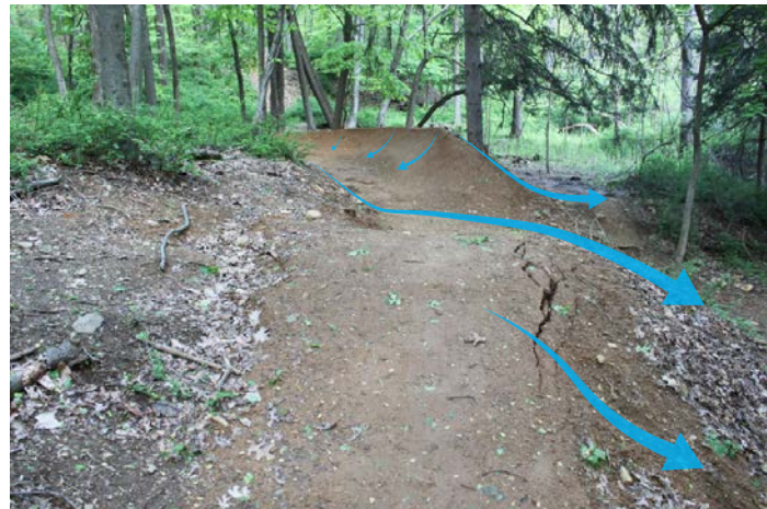
Determine the direction of flow onto, across, and off the trail
