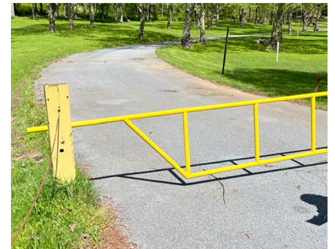
Permanently closed gates limit the ability of visitors to access large areas of the park conveniently.
